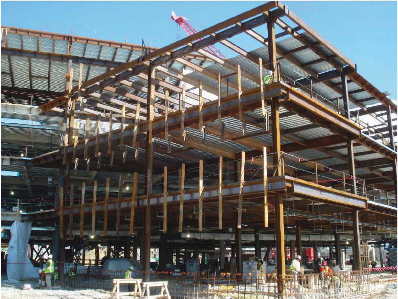
Curtain wall facade partially erected. Vertical HSS members in place.
