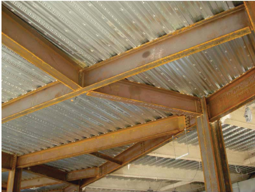
Typical erected "tie" beams
