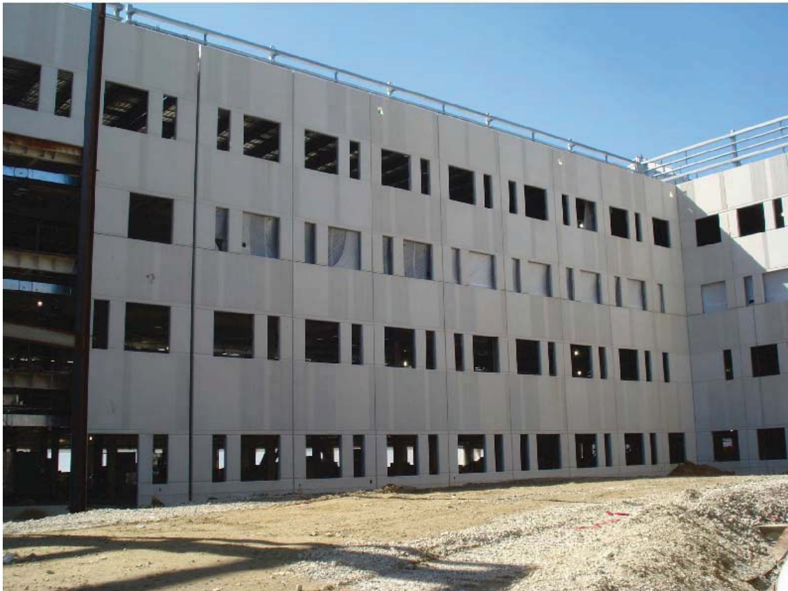
Erected Precast Panel facade in Courtyard
